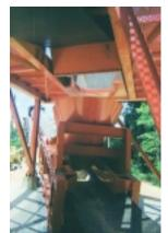
Figure 20 - Conveyor 6 to 7, 72-inch wide belt conveyor system, transfer point as it was being installed.
